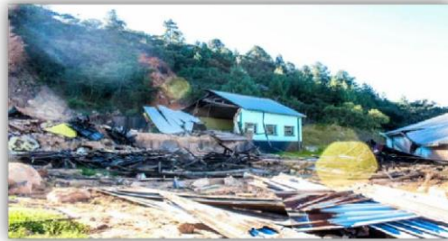
The remaining structure of the dining hall
