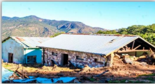
The damaged ablution facilities
