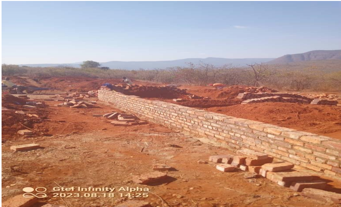
The foundation of a classroom block being constructed
